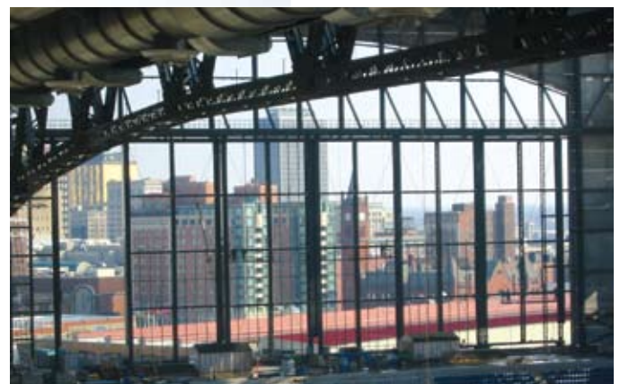
A view of the kinetic wall inside the stadium during construction
